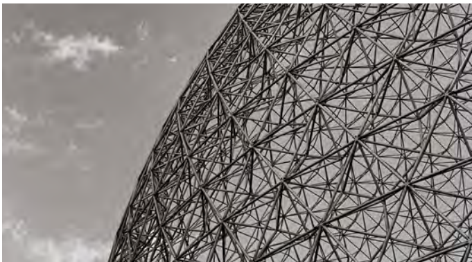
View of Buckminster Fuller's Geodesic Dome structural design of the United States Pavilion at the 1967 World's Fair.
