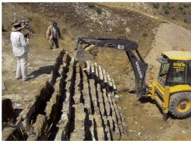
Conserving the stepped stone retaining wall of 8th century BC date at Gordion.
